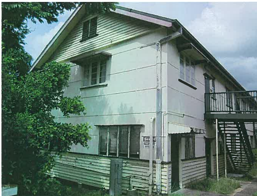
Image 16: Wall cladding around the outside of the building is asbestos cement sheeting.
