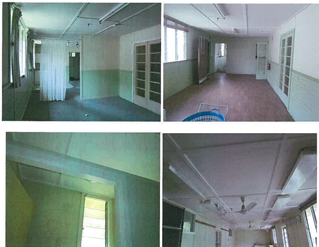
Image 7: Ceilings linings to all the lower side rooms are lined in asbestos cement sheet ceiling lining.
