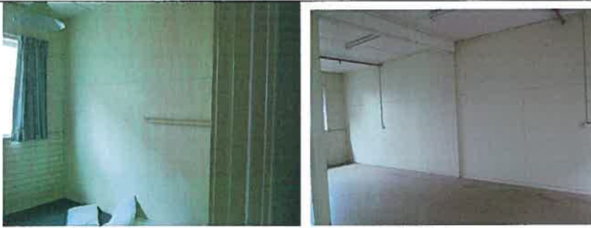
Image 20: Examples of the single panels or walls of asbestos cement sheeting.
